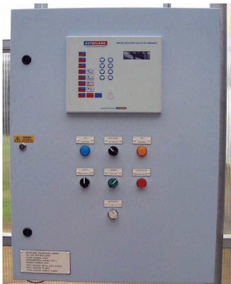
The biggest advantage of servo control is when it is coupled with a computer to control all the capabilities of a burner. For example, AutoFlame makes a control package that, when coupled with a fully modulating burner, can increase your boiler efficiencies 10-20 percent.
